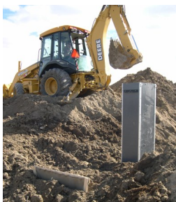
Water control structure being installed on connecting pipe between ponds.
